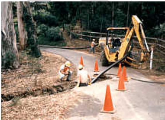
Figure A -3 Entry pit at lateral-to-mainline connection
