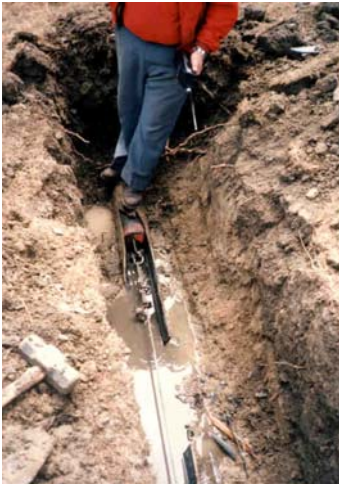
Figure A 6 Lateral pulling cable
