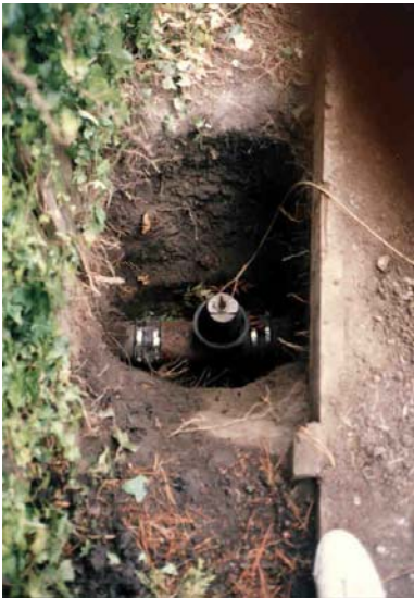
Figure A -8 Test plug in the lateral at the property line
