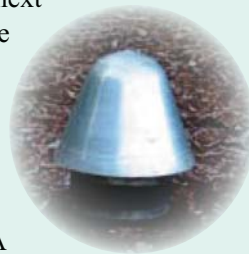
Mushroom type backflow prevention device
