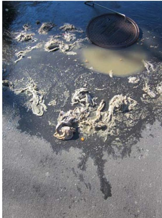
The picture above was taken after non-dispersing materials clogged a local sewer main, causing sewage to overflow onto a public street.
